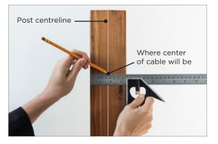
A3. Using a carpenter's square, measure and draw a line to the inside of the post face to find the center of your cable. Use the fitting as a guide to determine to centerline.
