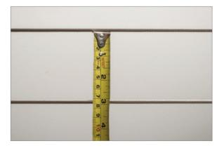
E2. Once all tensioners have been been tightened, test the cable run for deflection. Once all cable runs are properly tensioned the cable spacing should measure 3". The cable runs should be taut. The cable should not exceed a 1/2" deflection and a 4" sphere should not be able to pass between two cable runs. If more than 1/2" deflection exists, repeat step 12 until greater tension has been achieved. Do not over tension.
