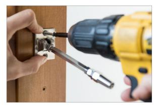
B2. Affix the Fastener Plate to the post with the two  $\#8 \times 1-3/4"$  stainless steel alloy 316 screws for wood posts.
