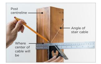
A6. Intermediate post: Determine the marked angle on the post. An angled jig (not shown) can aid in drilling on an angle to minimize errors. Drill at the marked angle through the intermediate posts to accept 1/8" cable with a 5/32" drill bit. Ensure that the drill holes are in line and at the same angle as subsequent intermediate posts before drilling. Remember to measure twice, drill once.
