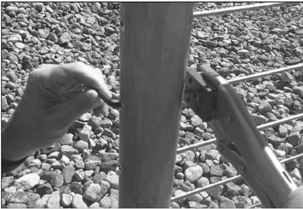
2. Tension all cables in sequence, beginning with the center cables, moving up and down toward the top and bottom. As you tension each cable, give it a sharp pull downward mid-span to help set the wedges, then re-tension as necessary in the same sequence. Be aware that the cable may move as much as 3/16" toward the tensioning terminal as the wedges seat.
